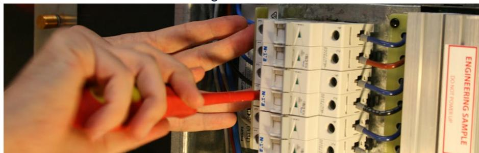
The control module installation is now complete. The lighting/load groups can be terminated into the module's output terminals.
