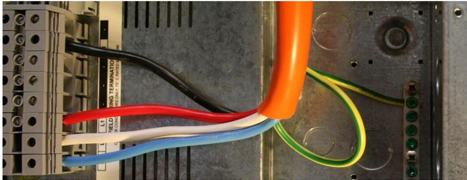
5. Terminate the supply group of the wiring loom into the left-hand side of the terminals. Refer to 2.4.4 Wiring loom for more information.
