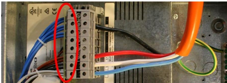
6. Recheck all terminal screws and tighten as needed.
