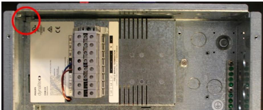
3. Secure the module using the fixing screw on the right. The unit should sit securely with no physical movement.
