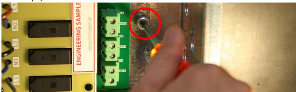
5. Terminate the control module's supply input wires into the right side of the circuit breakers.
