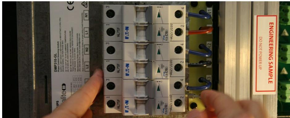
6. Terminate the corresponding Module group of the wiring loom into the left side of the circuit breakers.
