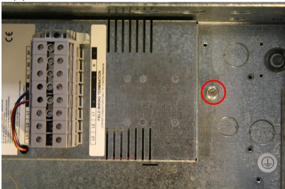
4. Terminate the supply wires into the right-hand side of the terminals and to the Earth bar on the right-hand side of the enclosure.
